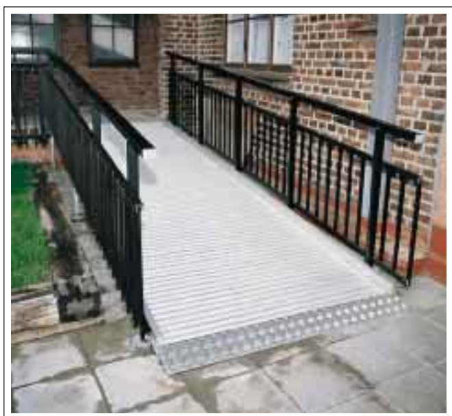
Gangway with intermediate balusters painted in black
