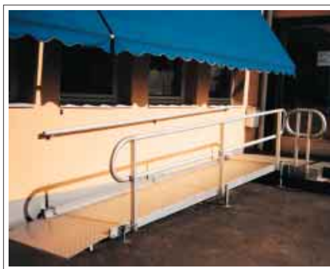
Gangway with landing, handrail fixed to wall
